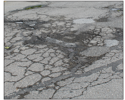
Parking lot at MS
