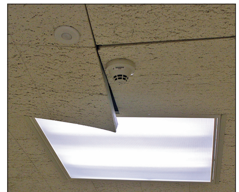
Ceiling at MS
