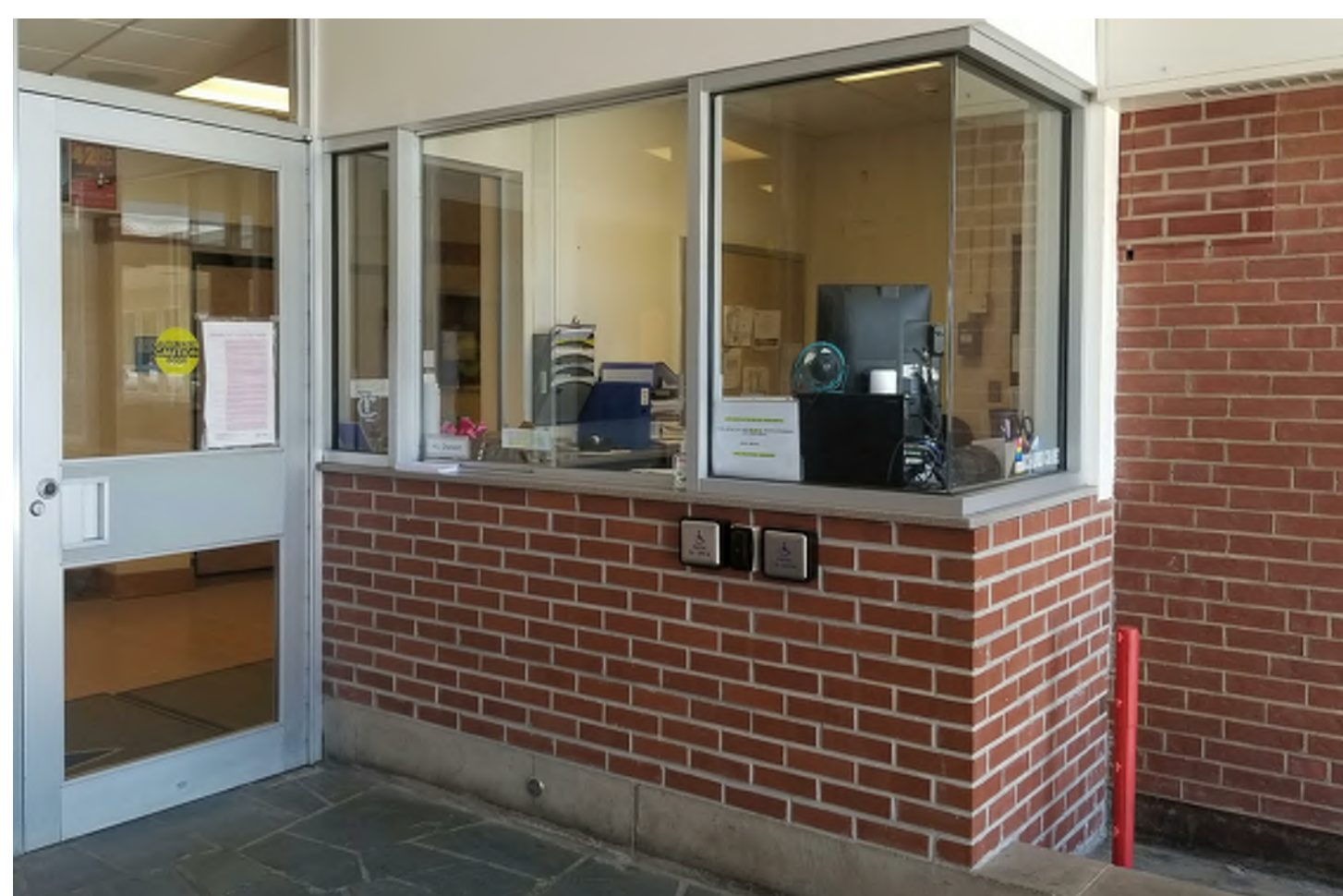
High School Vestibule Existing windows are open to intruders and easily compromised. Sliding windows would be replaced with fixed, bullet-resistant windows and surrounding doors/windows would receive impact-resistant film.
