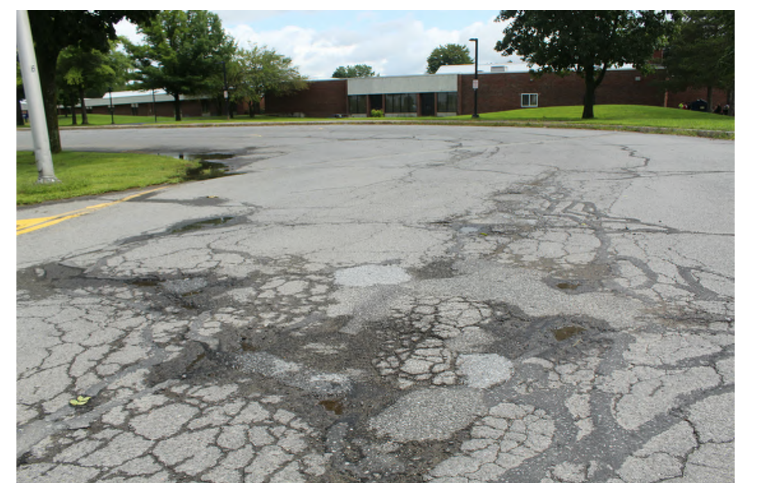
Middle School Entry Drive/Parking Lot Existing asphalt pavement is failing and in need of replacement. Pavement around the Middle School would be reconfigured to improve traffic flow and safety.
