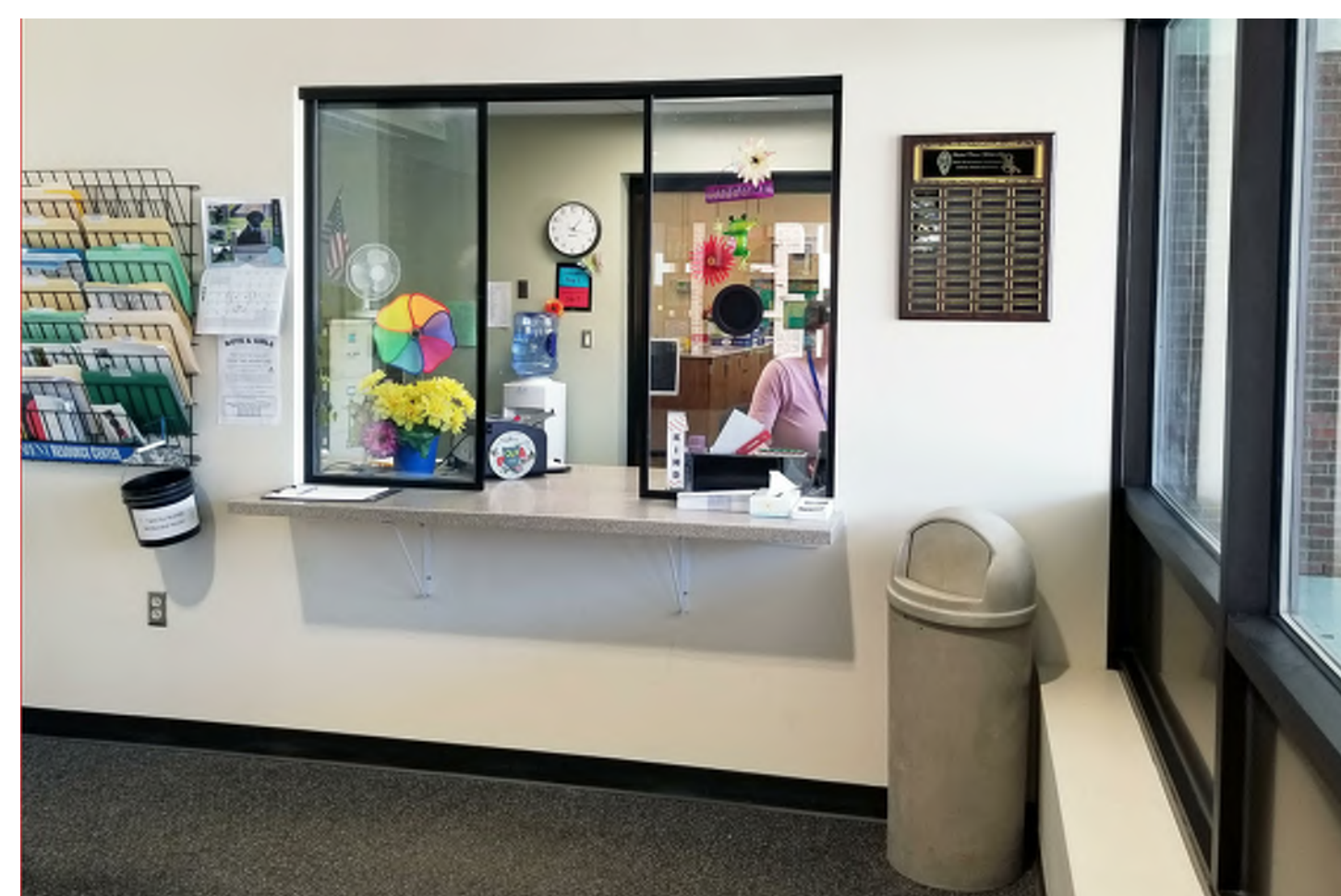
Middle School Vestibule Existing windows are open to intruders and easily compromised. Sliding windows would be replaced with fixed, bullet-resistant windows and surrounding doors/windows would receive impact-resistant film.
