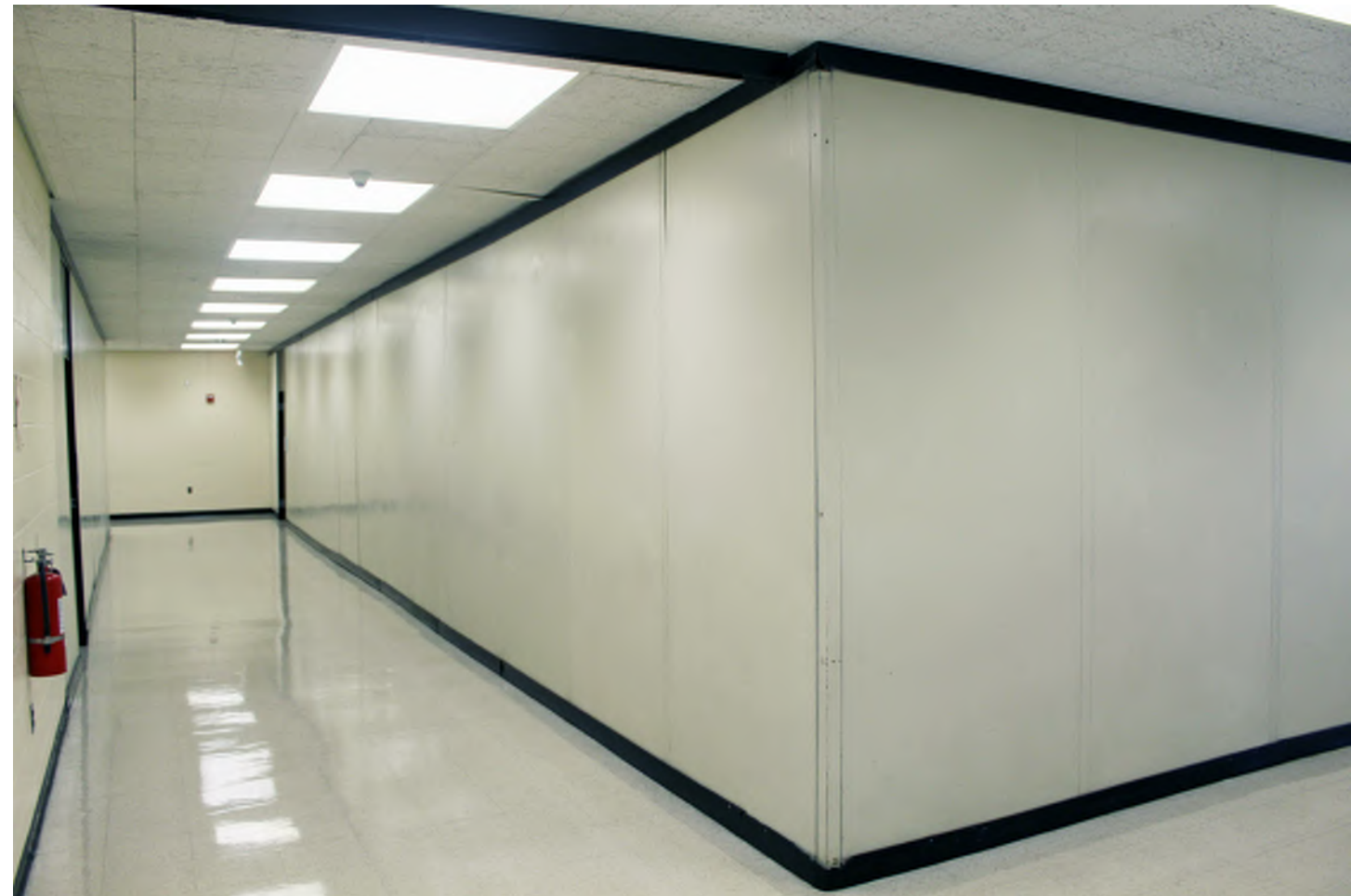
Middle School Classroom Partitions Existing classroom walls are temporary "dismountable partitions" which lack adequate sound separation and limit storage and electrical capacity. Safe & secure door operation within these walls is problematic.
