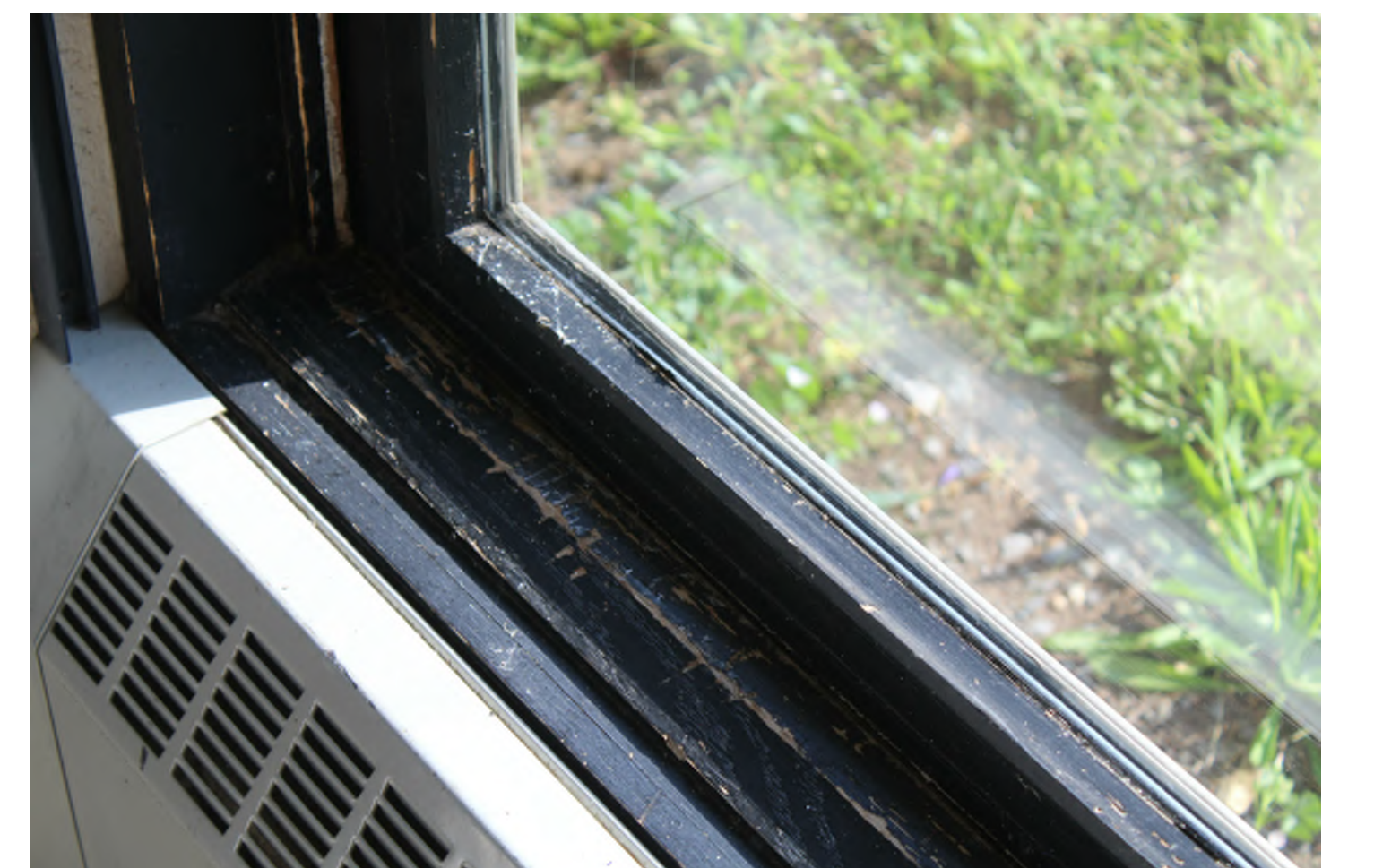
Middle School Classroom & Office Windows Existing windows are single-pane glass which offer no thermal protection. They have also begun to fail and allow water penetration.
