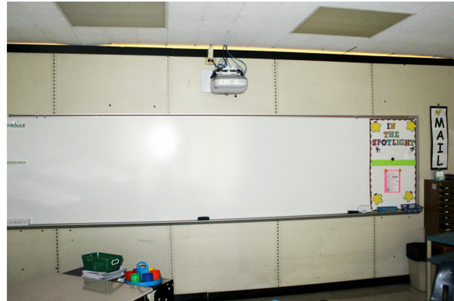
Middle School Classroom Partitions Existing walls run below ceilings, allowing for sound transmission between classrooms & corridor. New walls that extend to the underside of the roof would provide proper sound isolation between classrooms.
