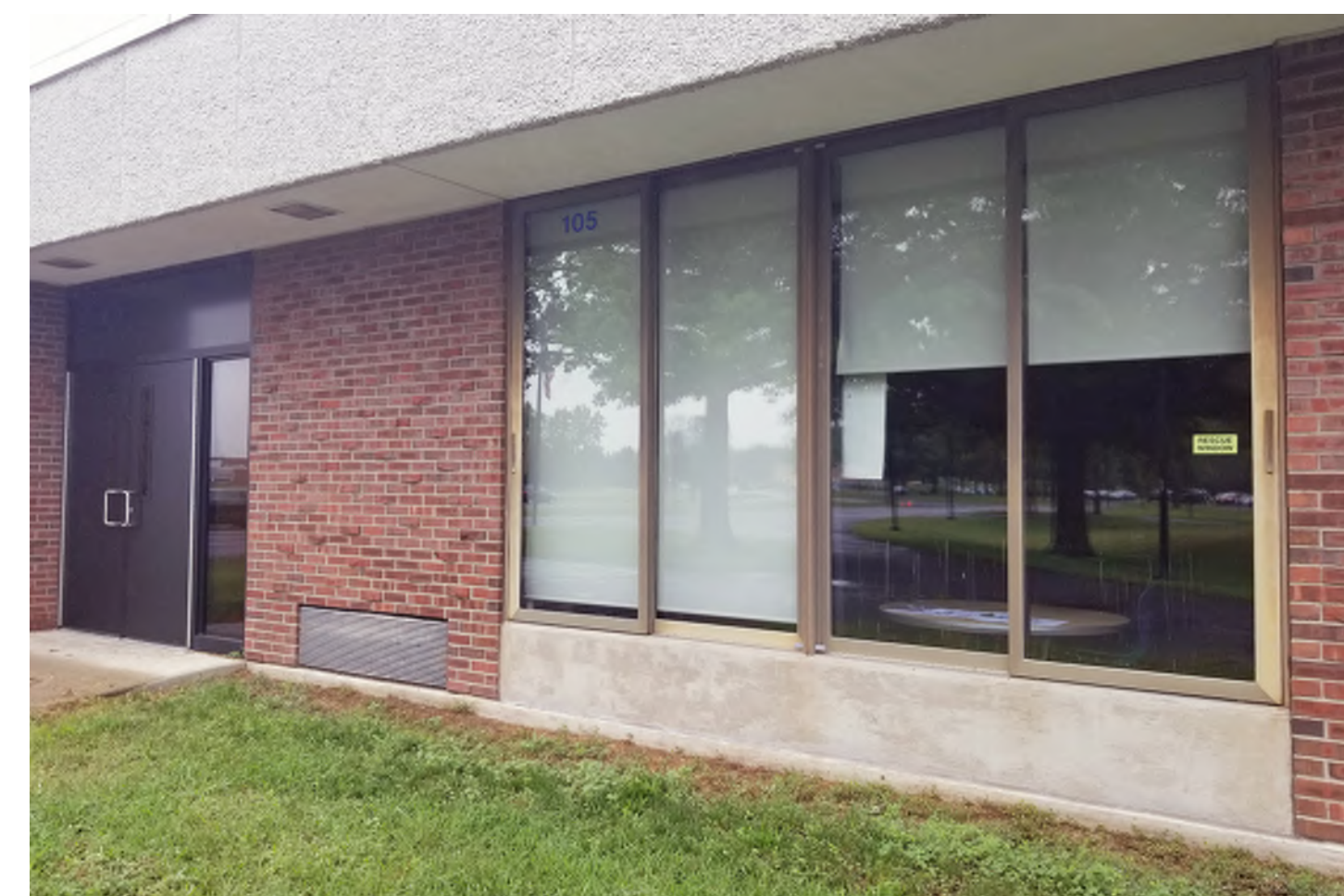
Middle School Classroom & Office Windows Existing windows are not energy efficient. Additionally, these windows are low to the ground and pose a security concern.
