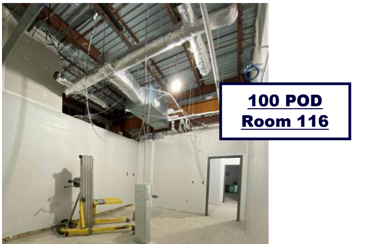
100 POD - Window Frame Install
